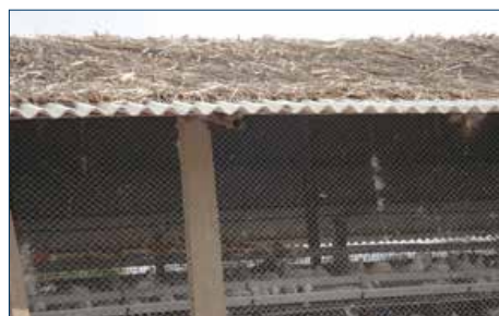
Figure 8. Use of thatching material (paddy straw, corn stalks, sugarcane tops) to reduce solar heating of the roof.
