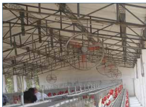
Figure 4. Stir fans and foggers increase air velocity within the house and create a cooling effect.
