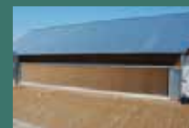
Cooling Pads & Fans
