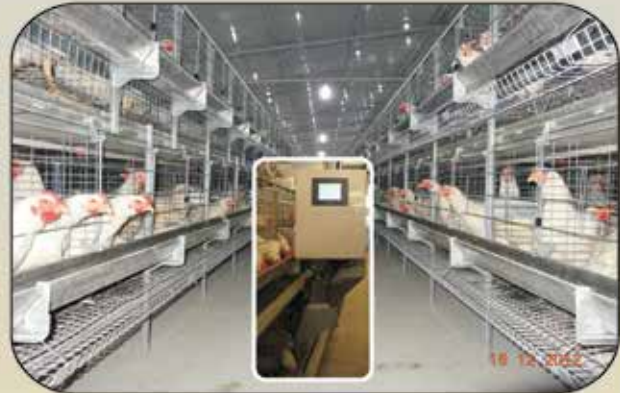
G E ULTIMA BATTERY FOR BROILER BREEDERS WITH ACCU-FEED WITH QDTS TECHNOLOGY FOR FEEDING
