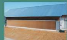
Cooling Pads & Fans
